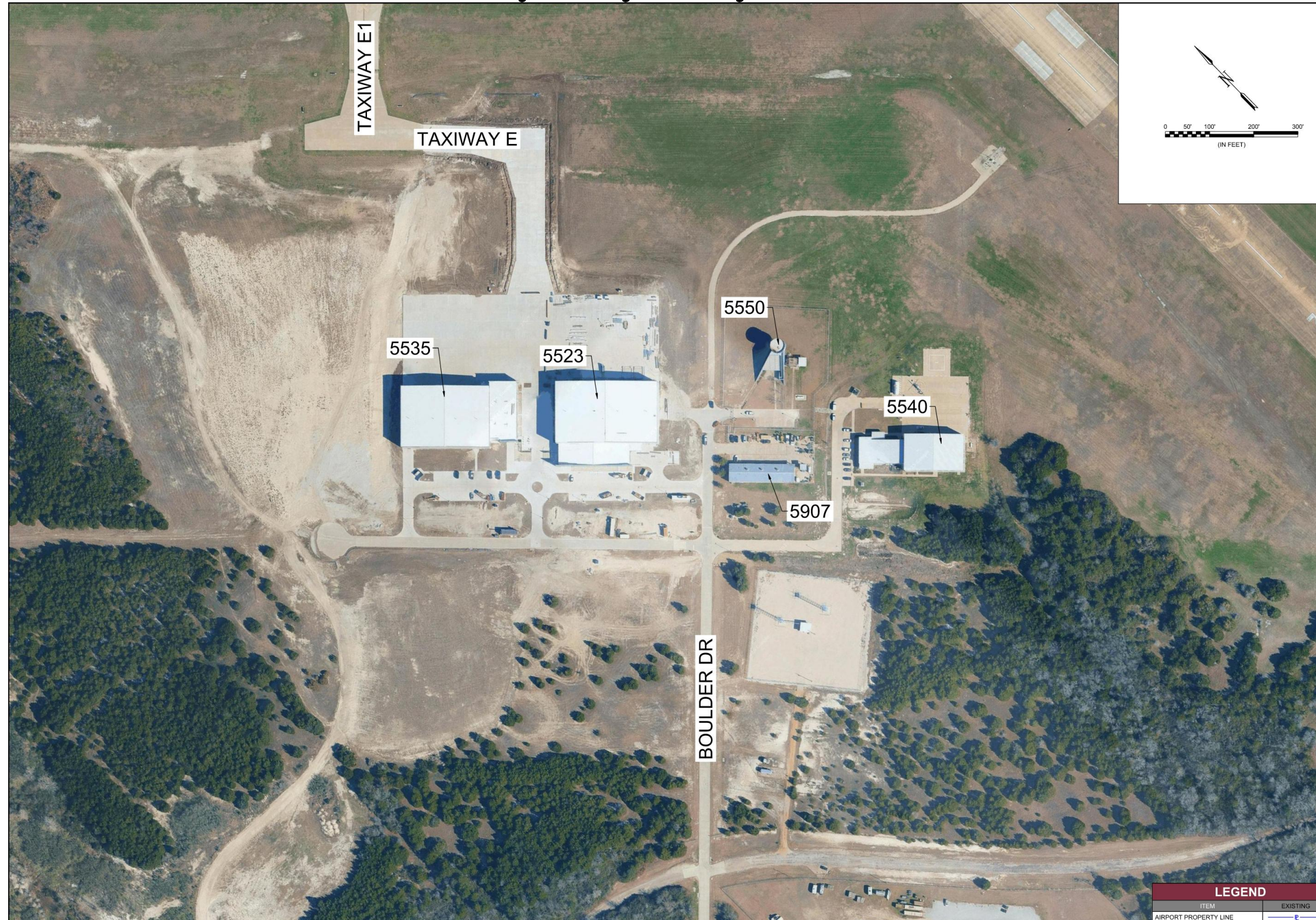
Figure 2-7 - Hangars and Buildings - Westside
