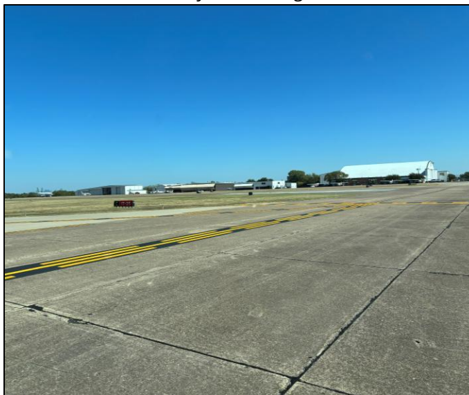
Taxiway C - Looking East
