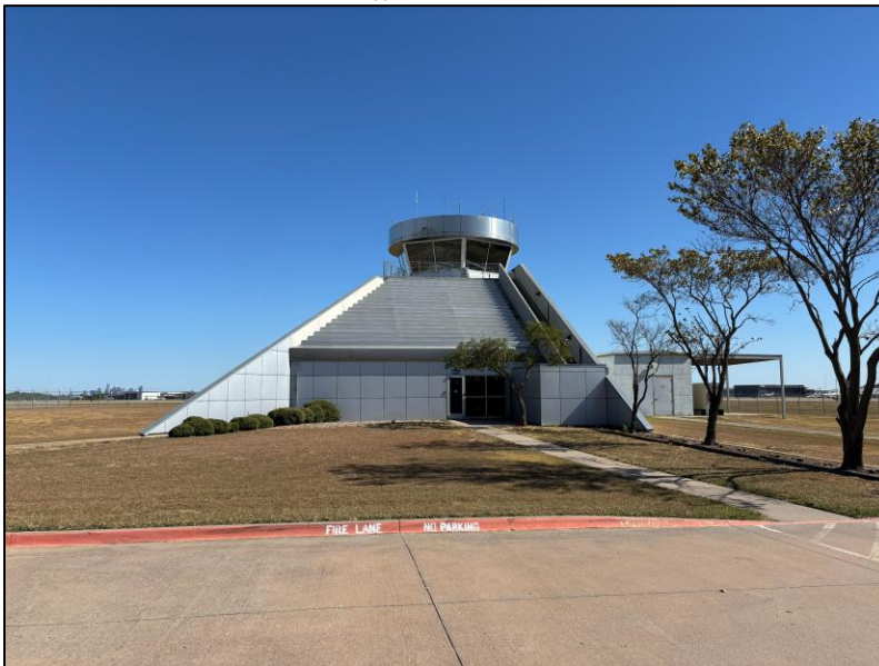
Air Traffic Control Tower
